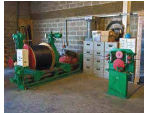
Cable cutting and re-spooling
